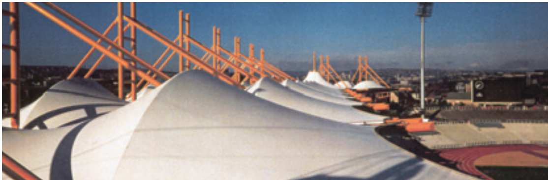
Stadium roofing over seating, Sheffield
